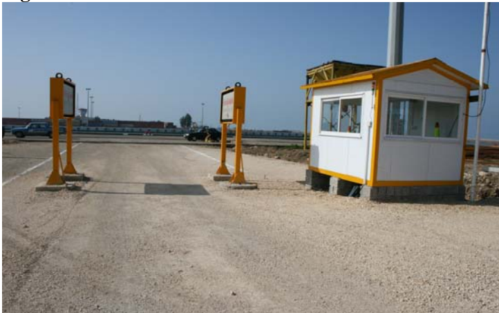
Fig 1. Portal Gate Monitor is installed at the borderline
